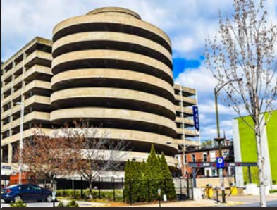
Spiral Deck 6814 W Linden Street Allentown PA 18101
